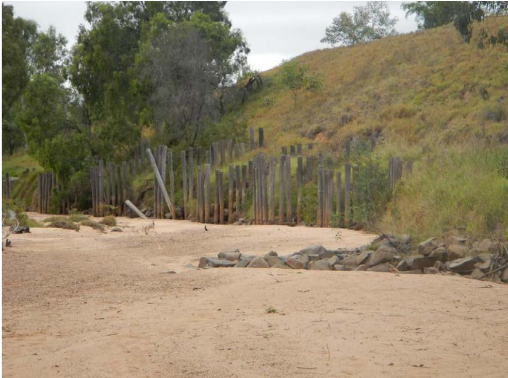
Figure 7.2 Example of Timber Piling
